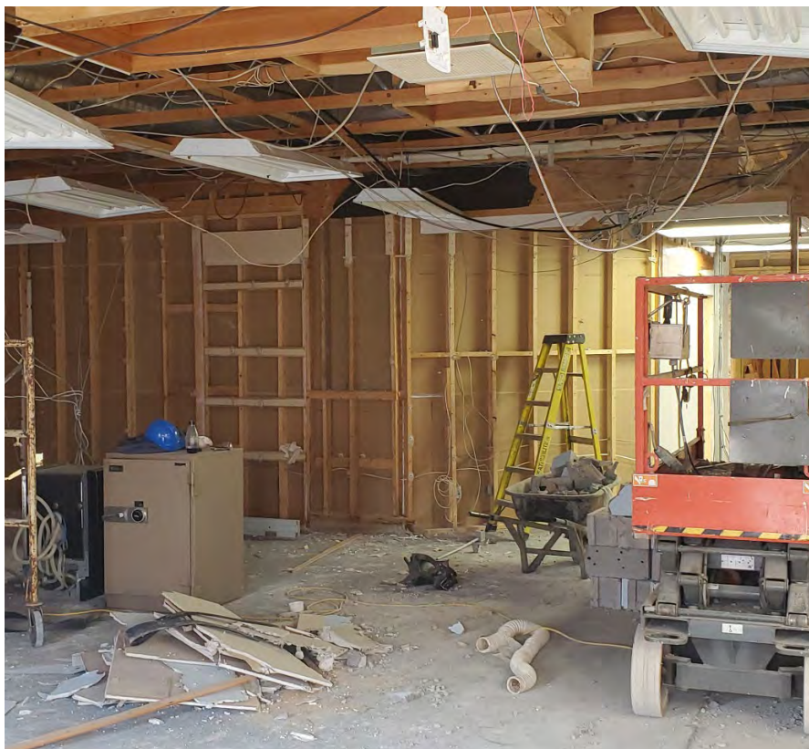
PHOTO: "Renovations on the Former District Office" by Tyler Madsen
